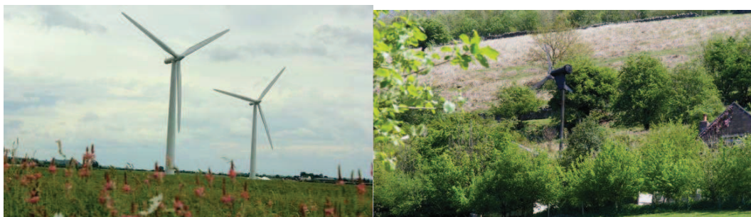
Figure 28, 1.3 MW Siemens (left) residential scale Proven turbine (right)
